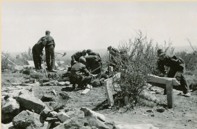
CCCers beginning work on the Park Point fire lookout, 1940. Courtesy National Park Service, Mesa Verde National Park.
