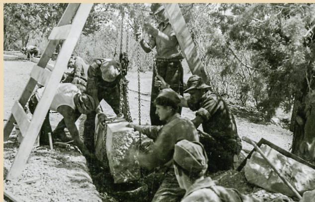
Rock from a nearby quarry being shaped for installation along the road at the park headquarters. Courtesy National Park Service, Mesa Verde National Park.
