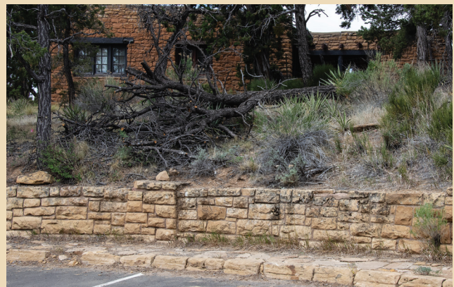
A CCC-built rock wall along the parking lot across from the Chapin Mesa Archeological Museum. Photo credit Todd Bacon.
