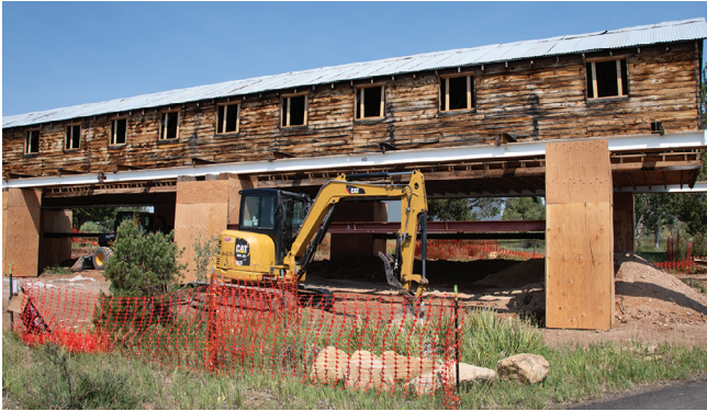
Barracks #5 getting a new foundation in 2024. Photo credit Todd Bacon.
