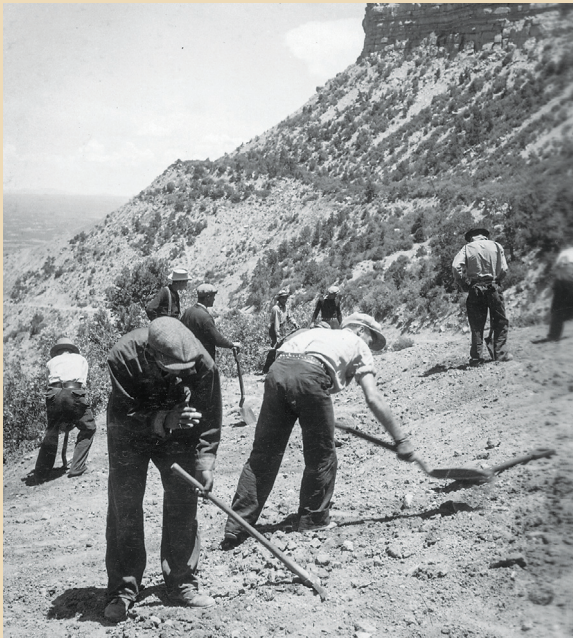
CCCers clearing a landslide on the Knife Edge Road. Courtesy National Park Service, Mesa Verde National Park.
